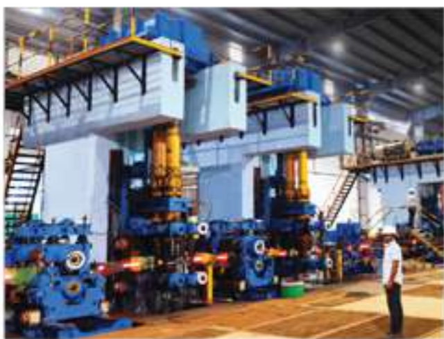
Rebar & Wire Rod Mills
